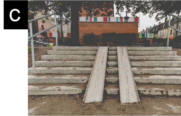
[Image description: Two thin, metal strips serve as a makeshift ramp with a flight of concrete, outdoor stairs between them.]
