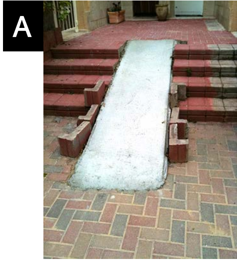
[Image description: A concrete ramp lays on top of a flight of stone outdoor stairs]
